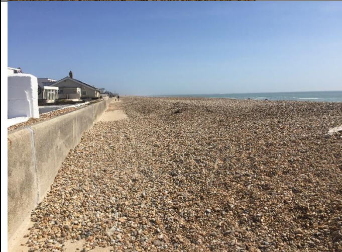
Photo 5: Shingle on the promenade at Eastoke Corner
