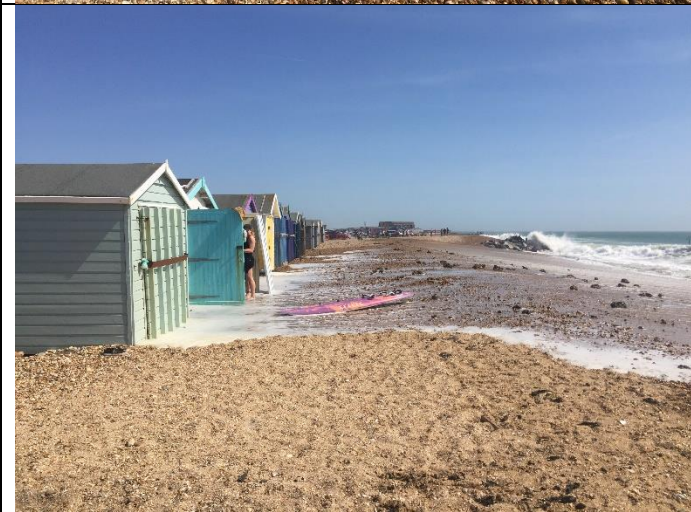
Photo 8: Flooding of beach huts and car park behind at West Beach, Hayling Island
