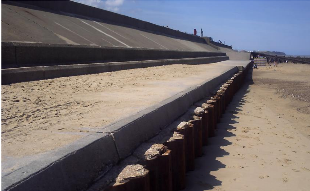
Photo 5: The sandy beach at Walcott, backed by sheet piling and concrete sea defence at EA survey transect N3C8 at Walcott in 2008. (Photo: Environment Agency)
