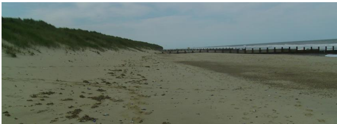
Photo 6: The beach at Horsey (EA survey transect N3A6) is backed by vegetated dunes and embankments, there are also timber groynes along this stretch of coast. (Photo: Environment Agency)
