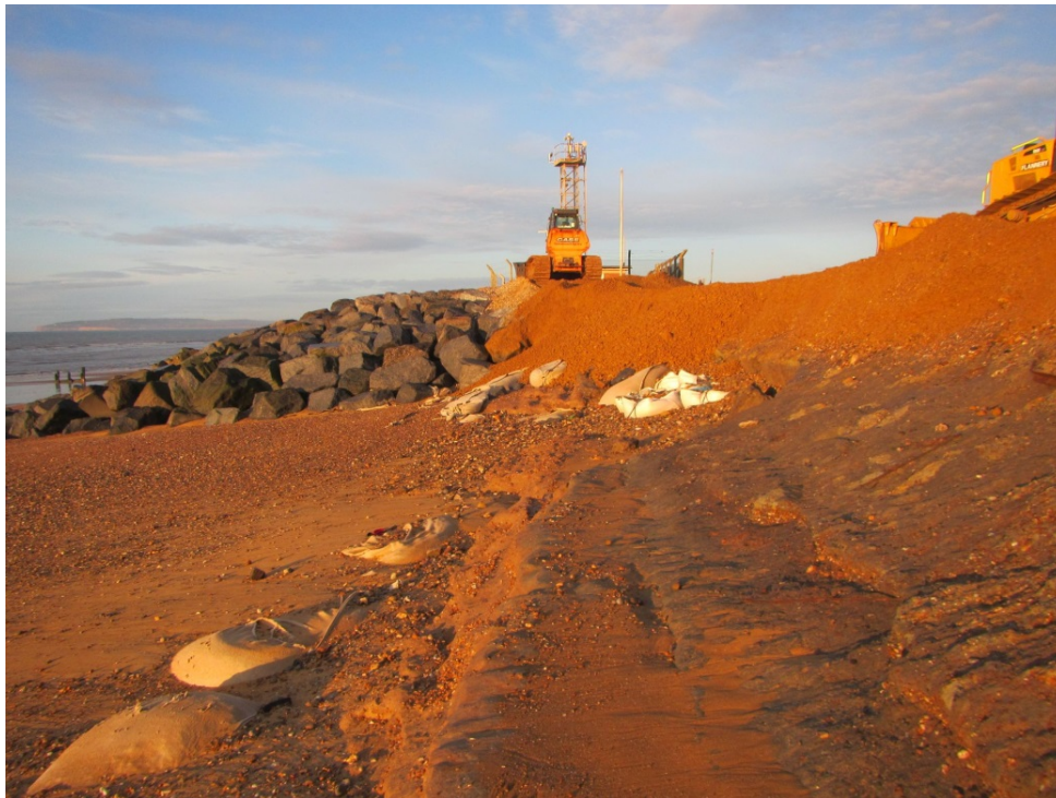
Figure 5- Depleted beach levels, geotextile bags have been exposed
