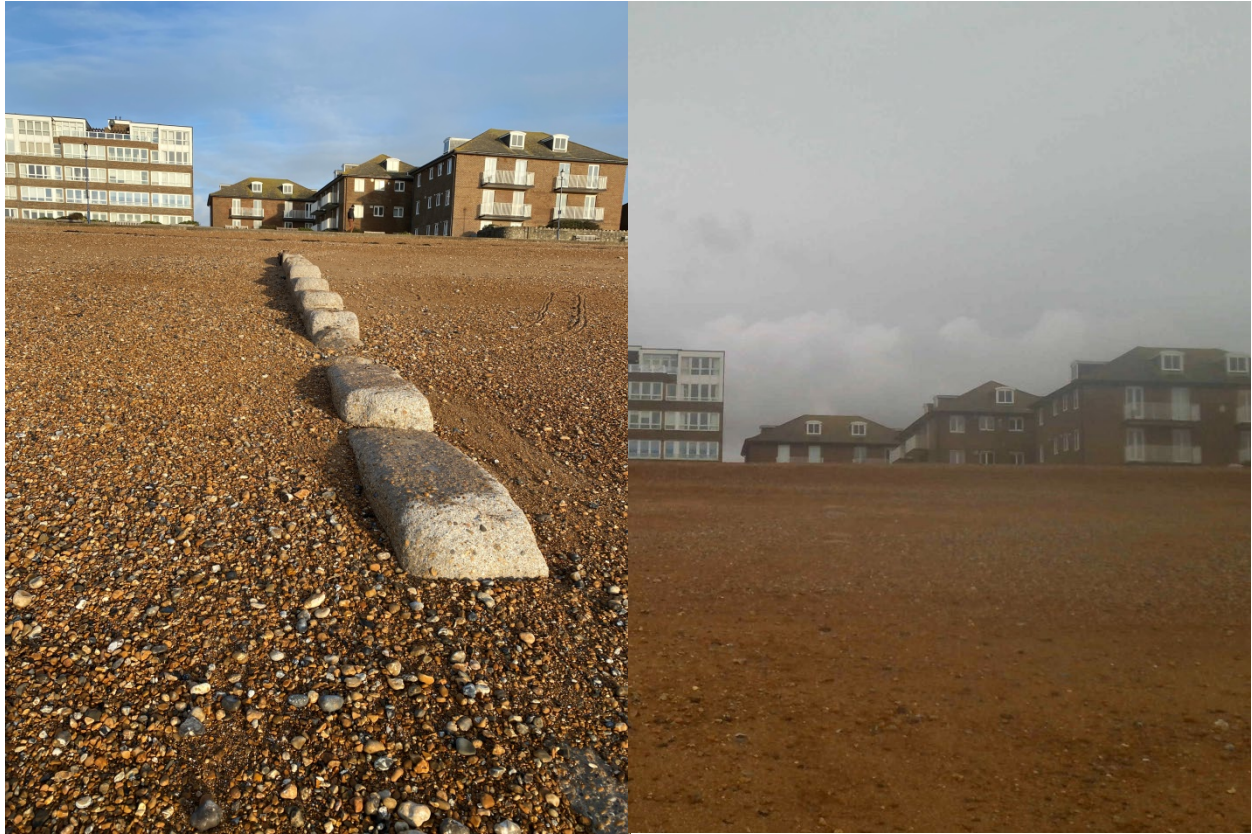
Figure 5 – Concrete groyne at Profile 4c00330, current (left) and October 2019 (right).
