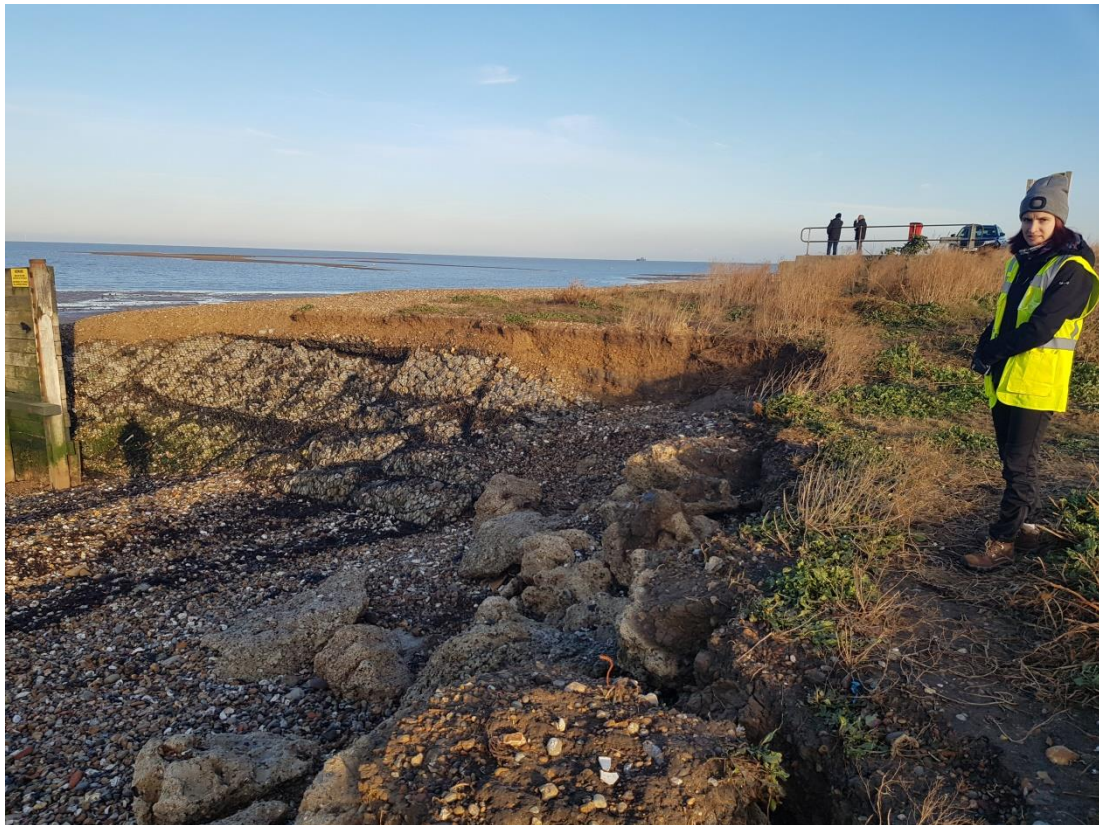
Figure 2.8- Exposed mattress and outflanked timber groyne at the Tankerton and Swalecliffe survey unit boundary.
